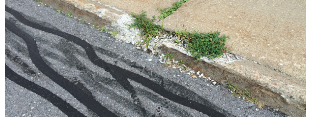
PDE pavement that will be replaced
